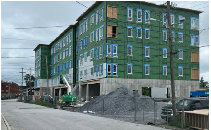
Construction site at Lake and Maple
