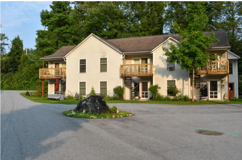
One of the existing buildings at Arlington Village Center. Courtesy of Shires Housing
