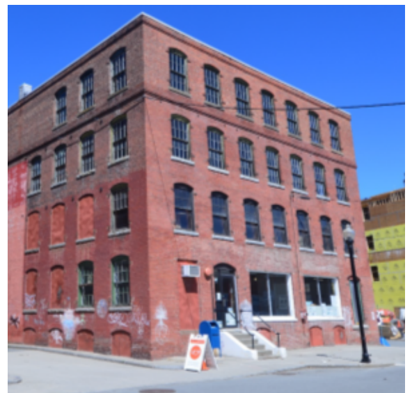
DeWitt Building in Brattleboro
