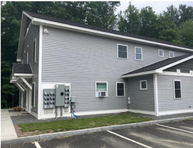
Photo of the completed building at Gordon Lane. Courtesy of Evernorth/Lamoille Housing Partnership
